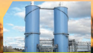
Dry Storage Tanks
